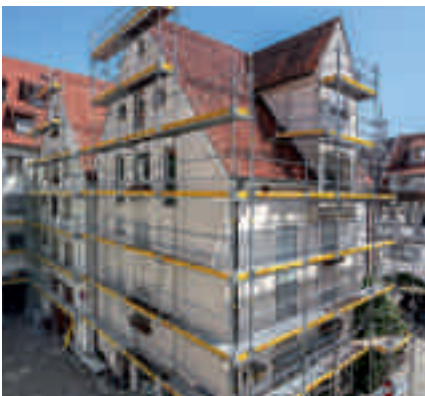
Renovation of an apartment building, Ulm, Germany
