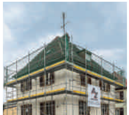
House renovation, Landau, Germany
